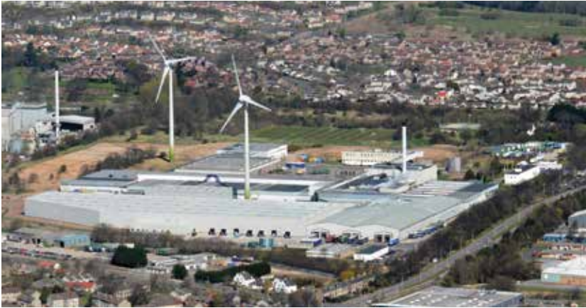
Two wind turbines supplying electricity to the Michelin tyre factory in Dundee.
