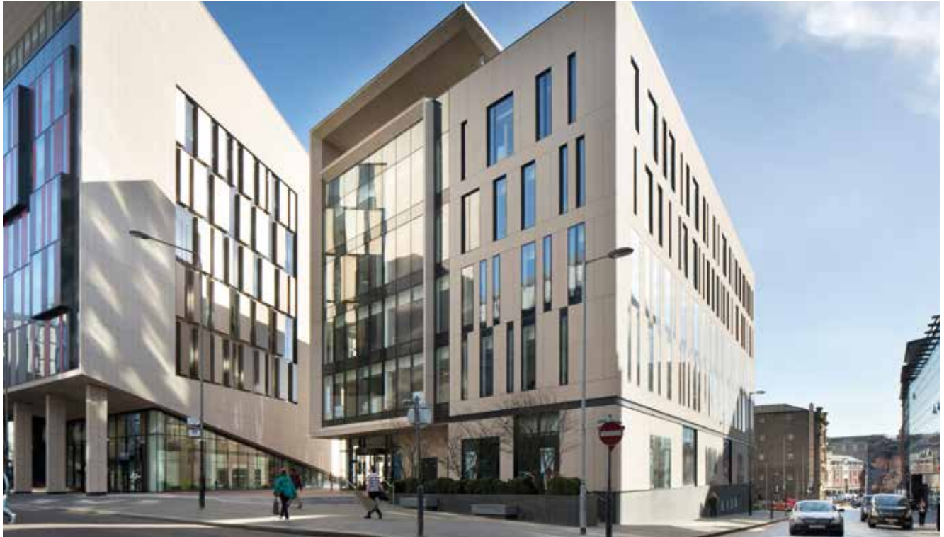
Exterior view of Inovo at ITREZ (International Technology and Renewable Energy Zone), Glasgow. Credit: Alan McAteer for Scottish Enterprise
