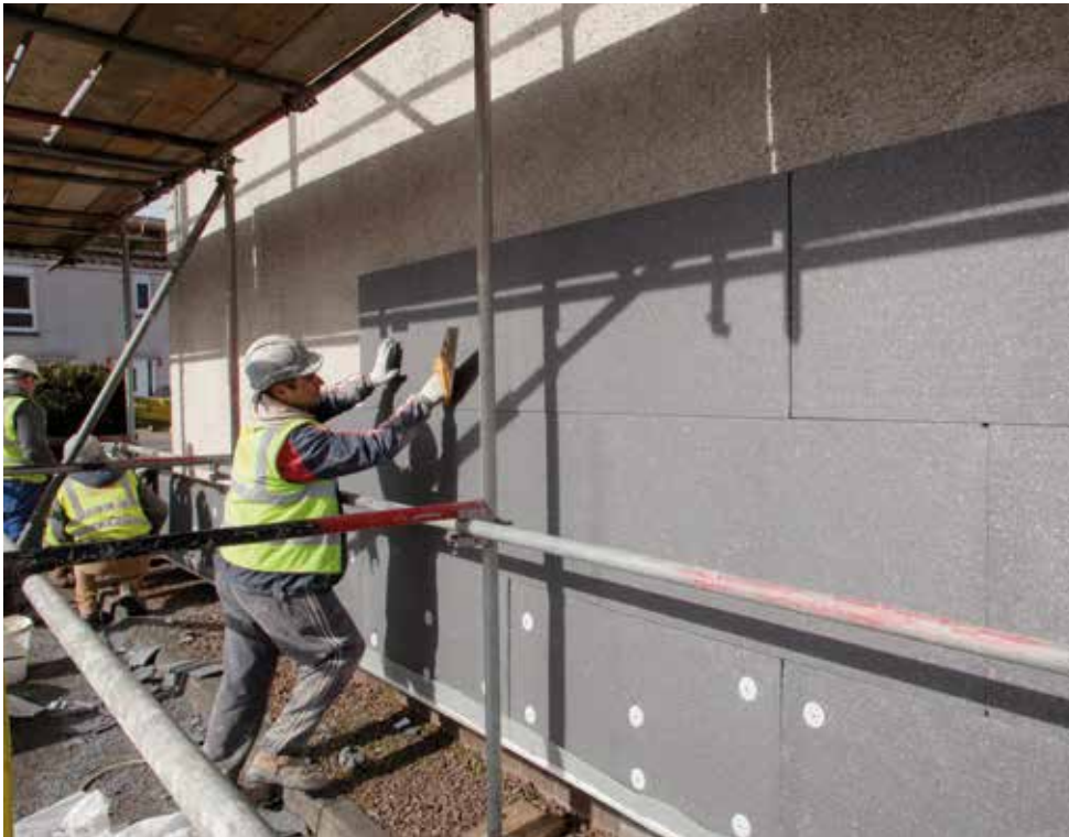
External wall insulation in Dunfermline.
