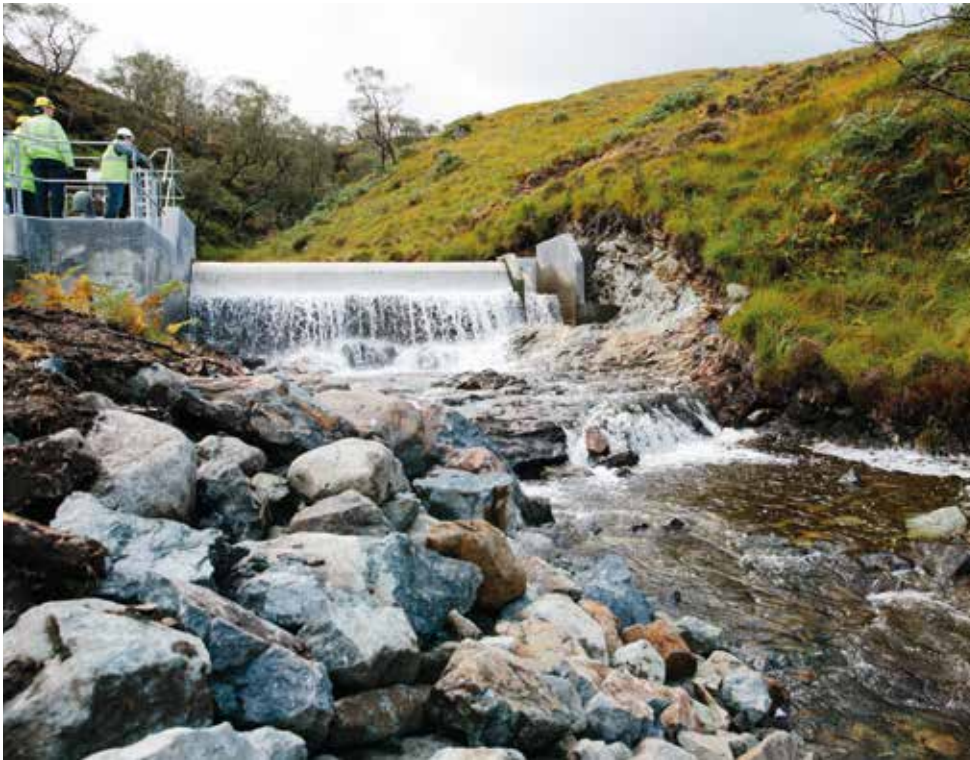
Garmony hydro scheme.
